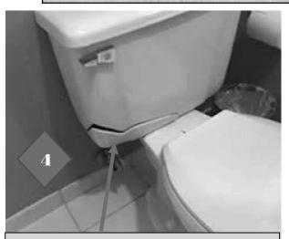
A cracked tank or dislodged flapper may not be detected for hours and can cause tens of thousands of dollars in flooding and water waste.
