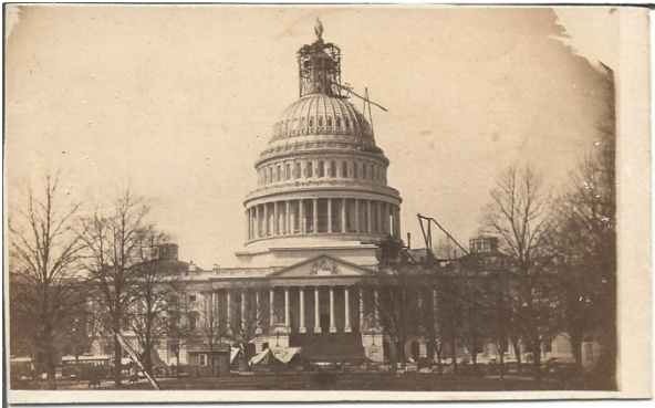
A View of the US Capitol Building Under Construction
