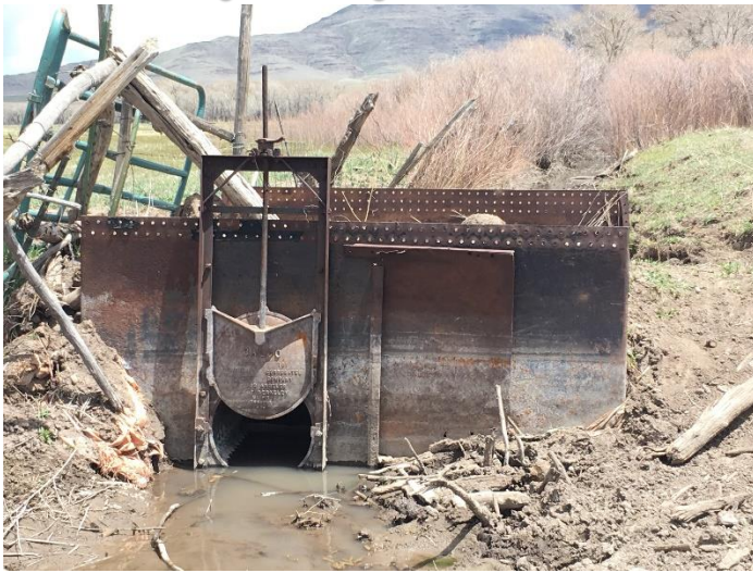
Headgate looking downstream
