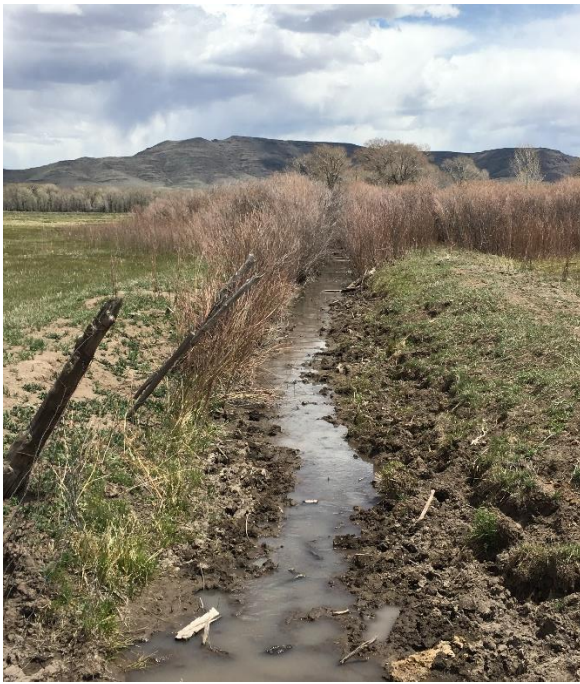
Ditch looking downstream of headgate
