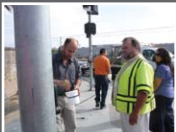
DPW, City of Chula Vista, CA
