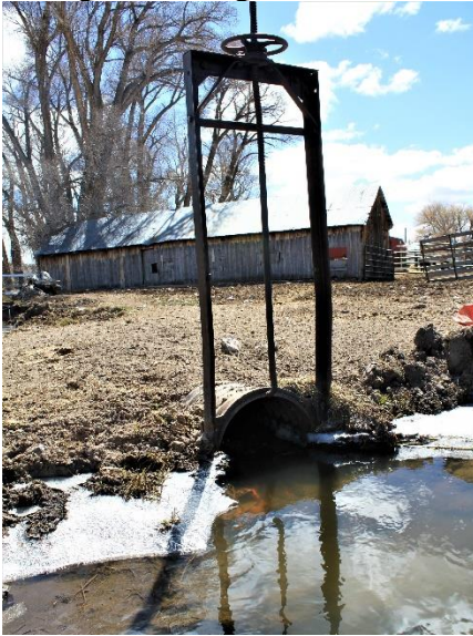
Headgate looking downstream
