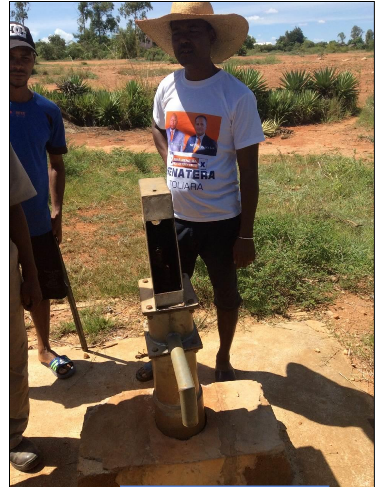
Broken Indian pump in Anambinda
