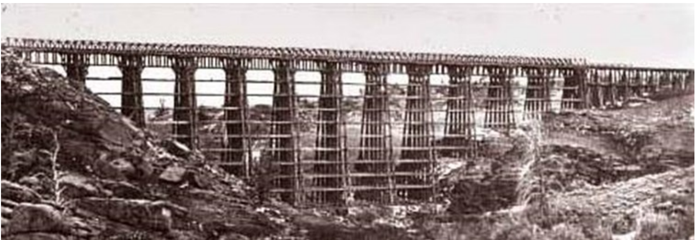
Dale Creek Trestle Bridge 1858 150 feet high and 650 feet long. It was twice replaced with steel.
