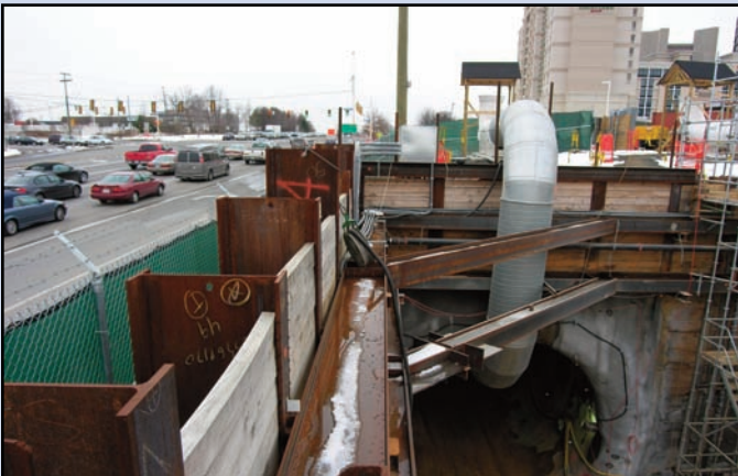
The inbound tunnel construction located directly next to the green fence along Route 123 near International Drive. Photo by Dulles Corridor Metrorail Project
