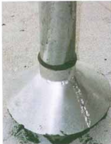
Sealant in caulk trough, located at bonnet of penetrating flashing
