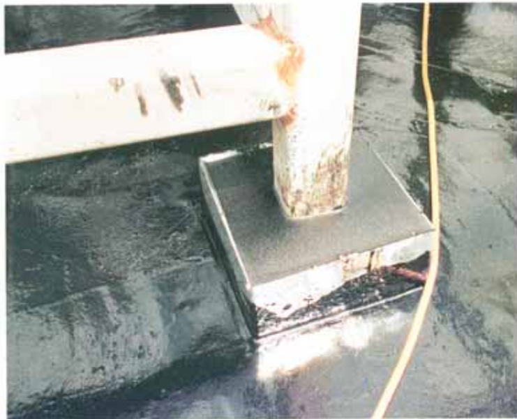
Pourable filler in pitch pan.
