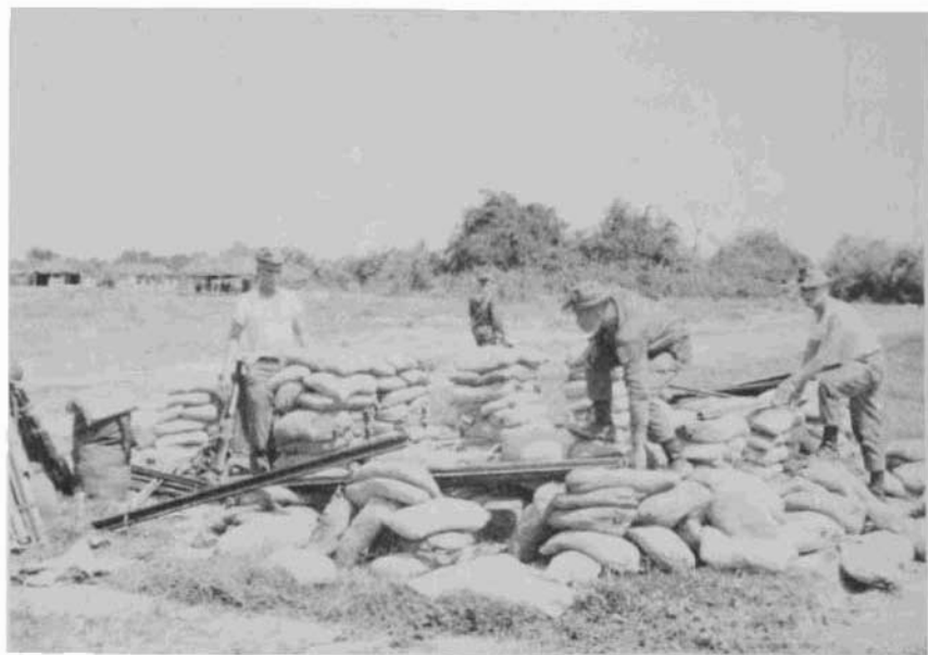
PHILIPPINE SECURITY TROOPS REBUILD A BASE CAMP BUNKER
