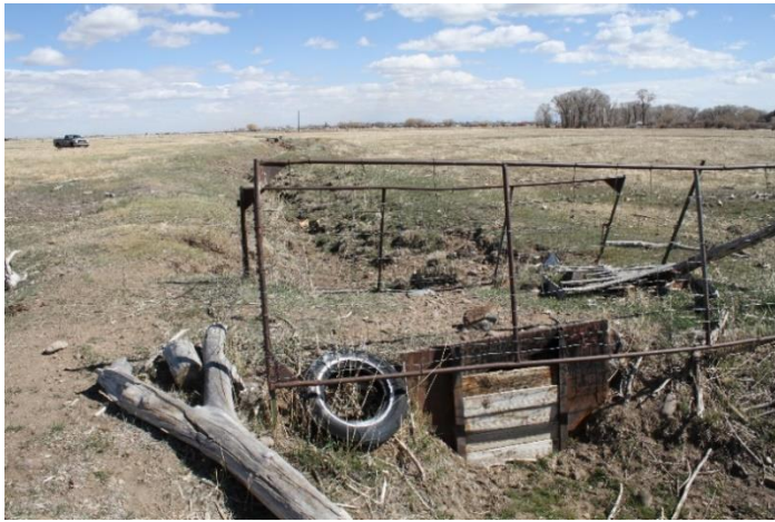
Headgate looking downstream
