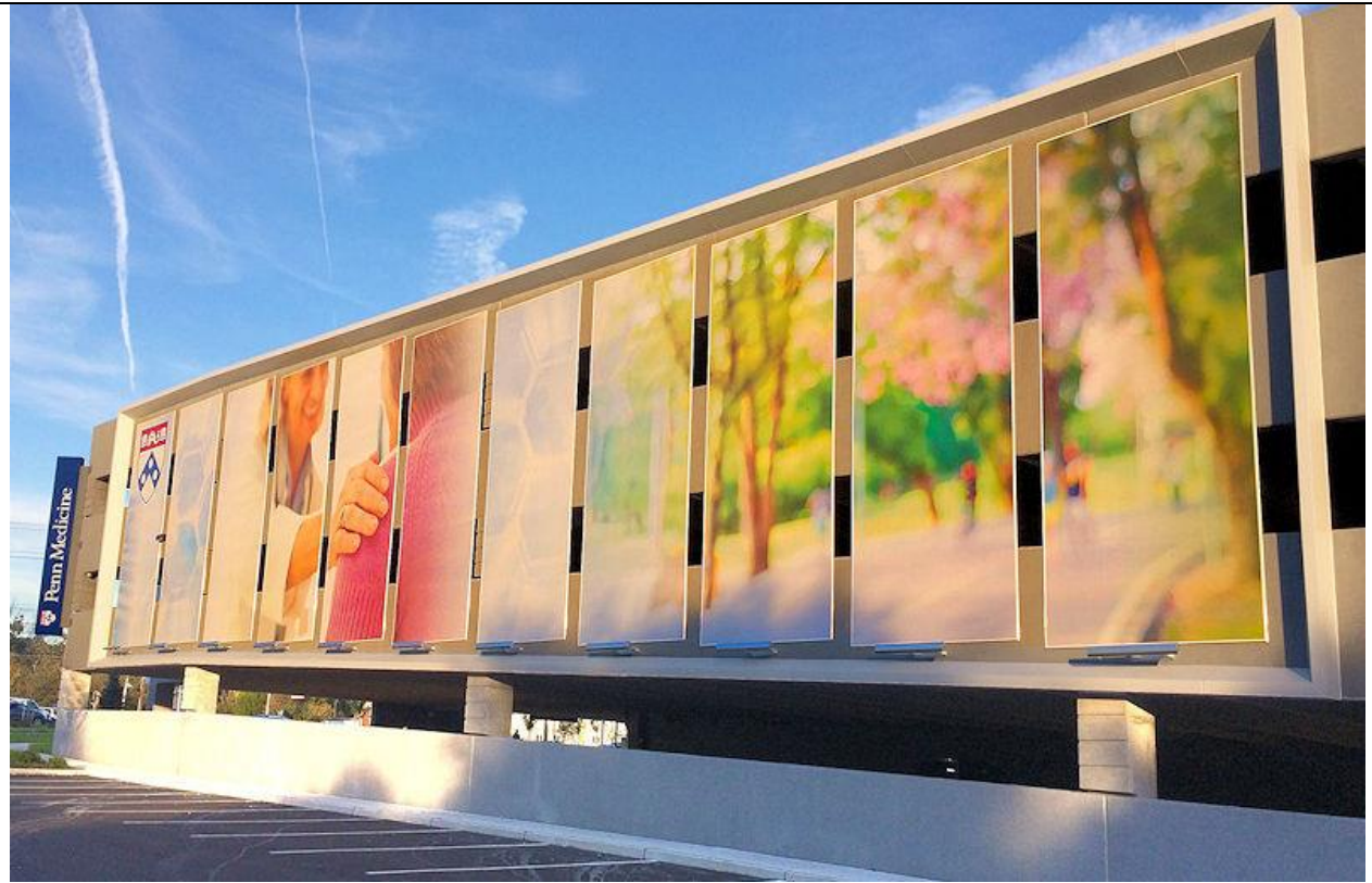
TS32 - Eleven 10ft x 24ft Banners stretched on a parking side We can see that the White PVC inserted on the side is discrete.
