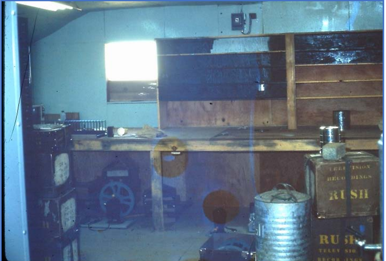
The Production Area Under Construction.
