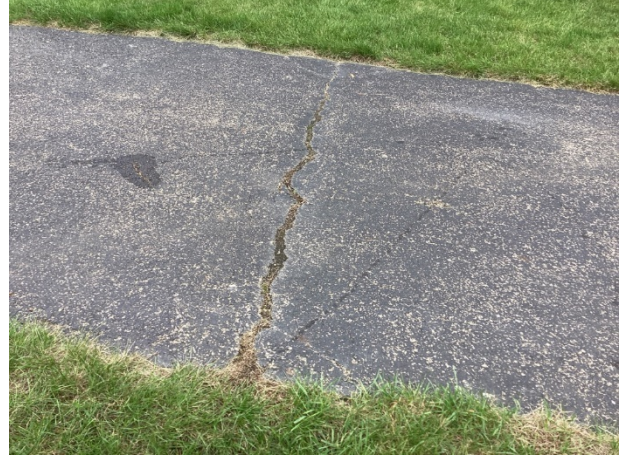
Transverse crack
