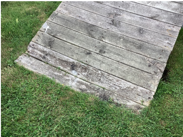
Weathered deck boards at small dock
