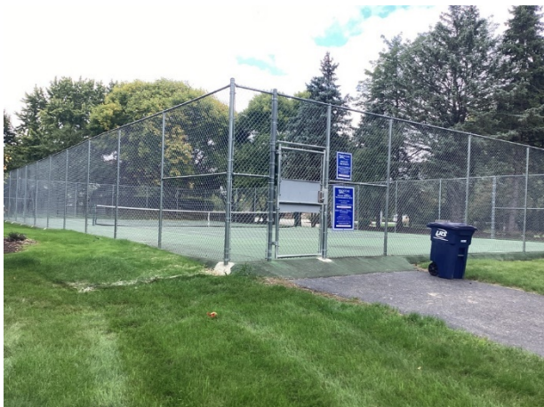
Chain link fence at tennis court
