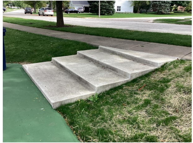
Concrete stairs at pickleball and basketball courts
