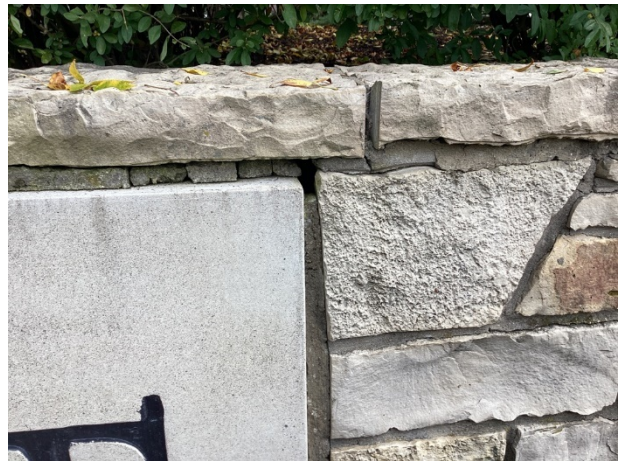
Mortar deterioration
