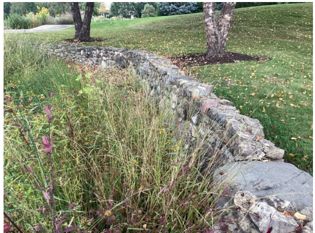
Mortar-set stone retaining wall
