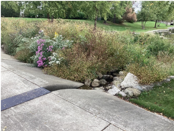
Rip rap and vegetation buffer zone between spillway and channel
