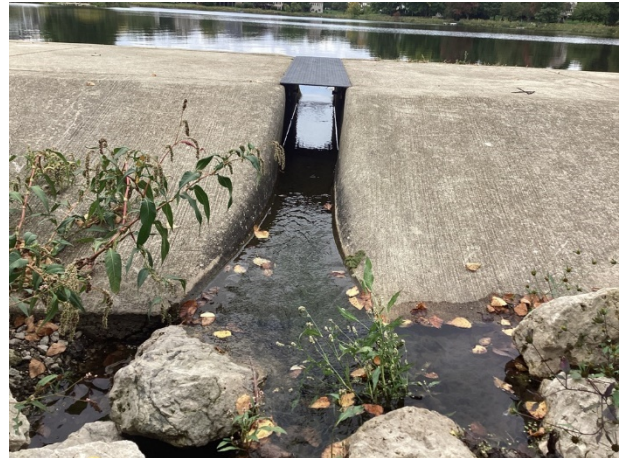
Spillway opening with metal cover
