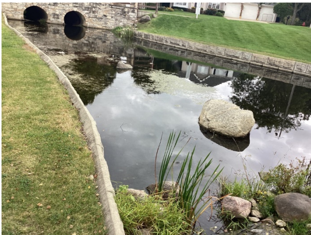
Algae growth at channel
