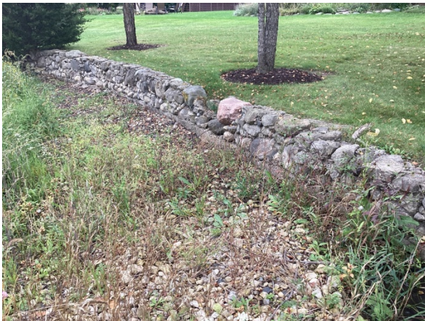
Mortar-set stone retaining wall
