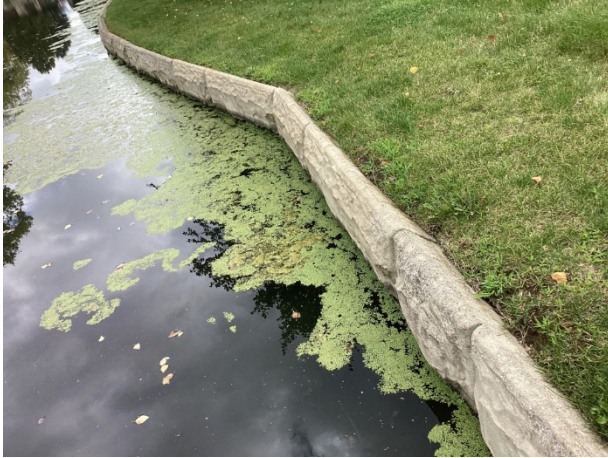
Concrete retaining wall
