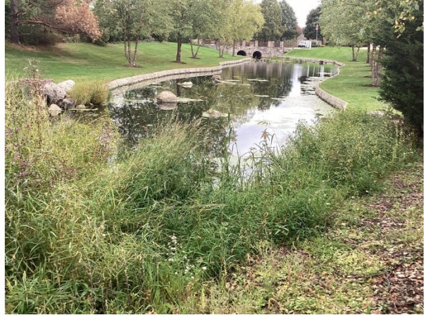
Channel downstream of spillway
