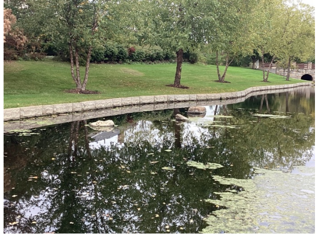
Concrete retaining wall
