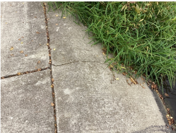
Concrete crack
