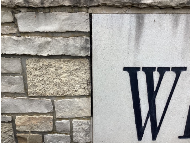
Missing mortar
