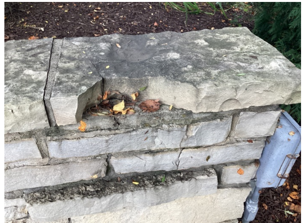
Masonry cracks
