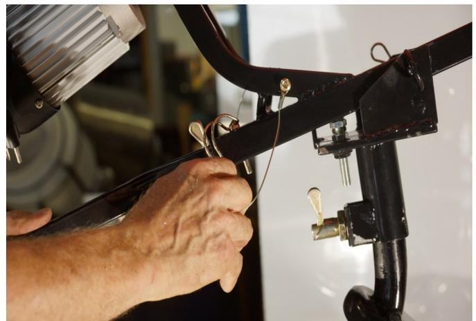
**Step 17**—Install handles attach with spring clip. Note, the handle can be placed in either the front position or the rear position for dumping.
