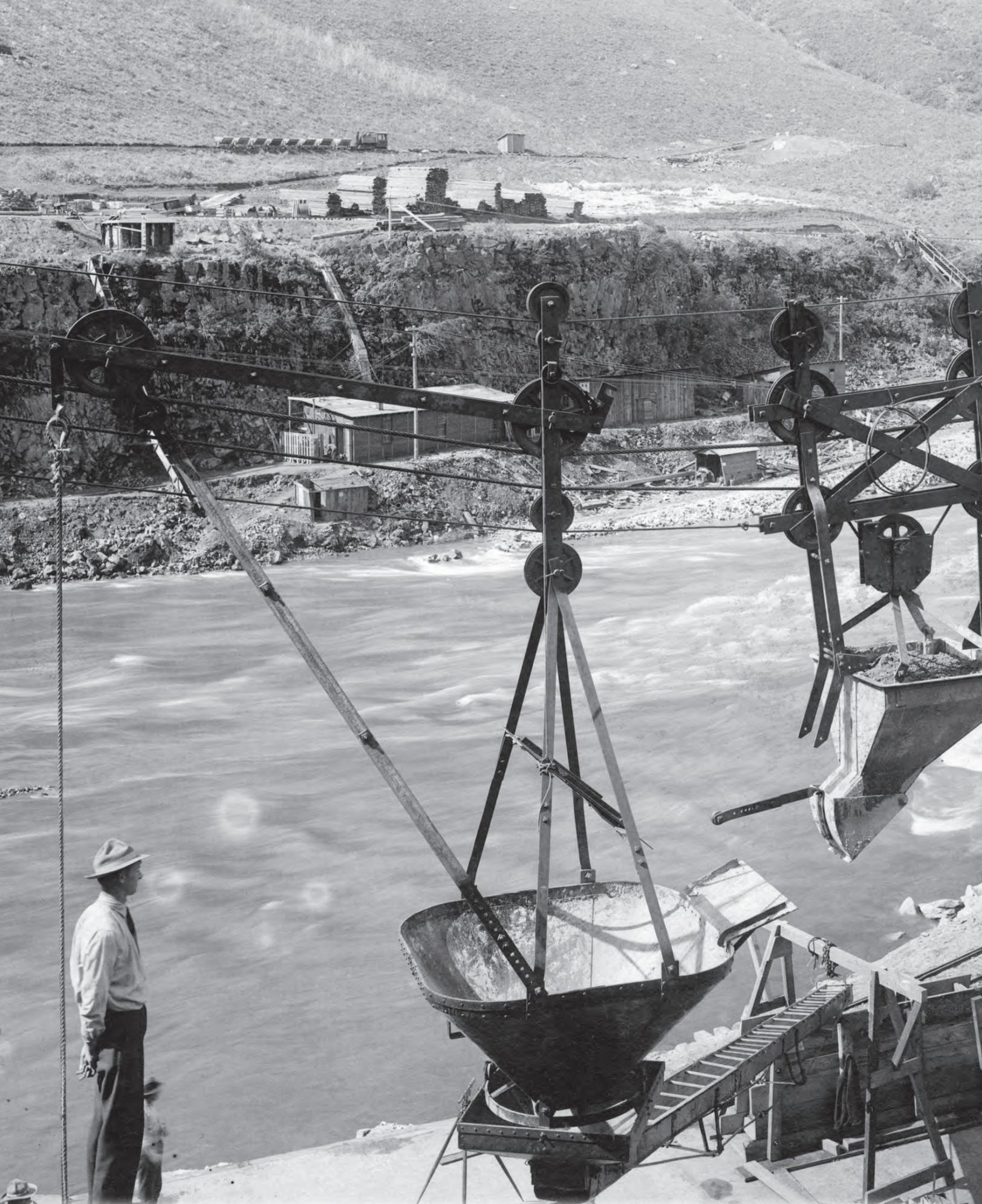
Arrowrock Dam, Crowe concrete distributing device about the discharge into the hopper. May 22, 1912
