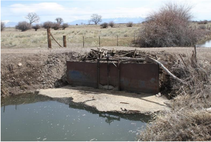
Headgate looking downstream
