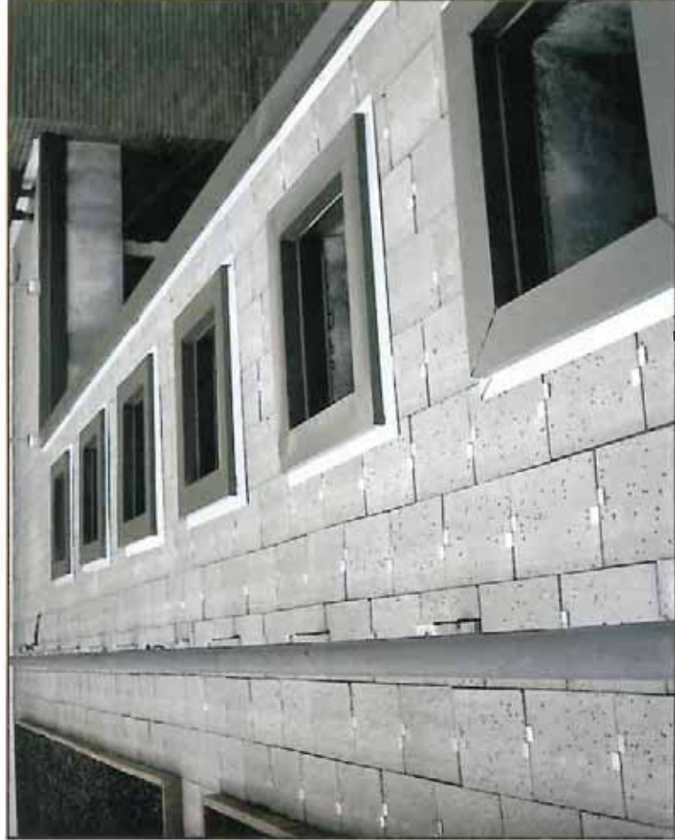
Typical perimeter paver condition.
