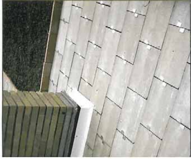
Typical wall flashing.
