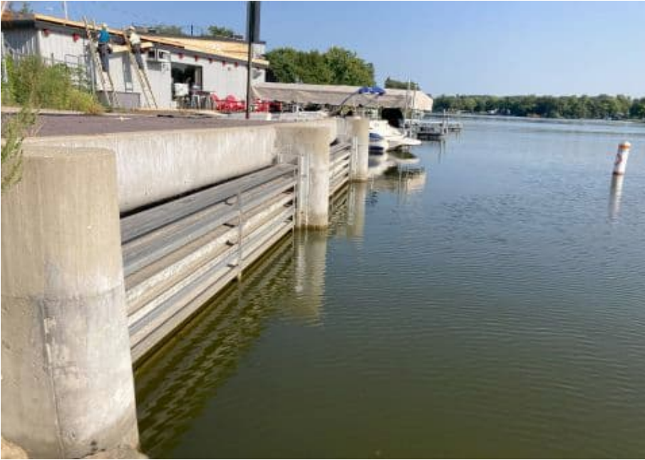
0011409092451 Stop logs at South Dam box culverts
