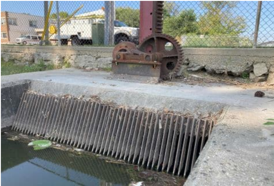
0011409092459 Looking D/S at South dam powerhouse headrace trashrack
