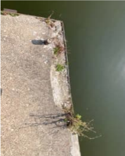
0011409092439 Chipped concrete on North dam LT U/S abutment
