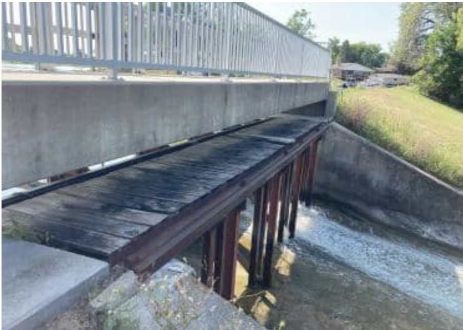
0011409092424 Looking south at North dam LT D/S abutment from RT D/S abutment. Old catwalk and stoplog frames visible between gates
