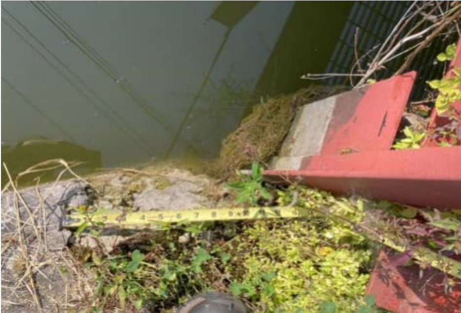
0011409092467 Spalling concrete on South dam RT U/S powerhouse headrace abutment
