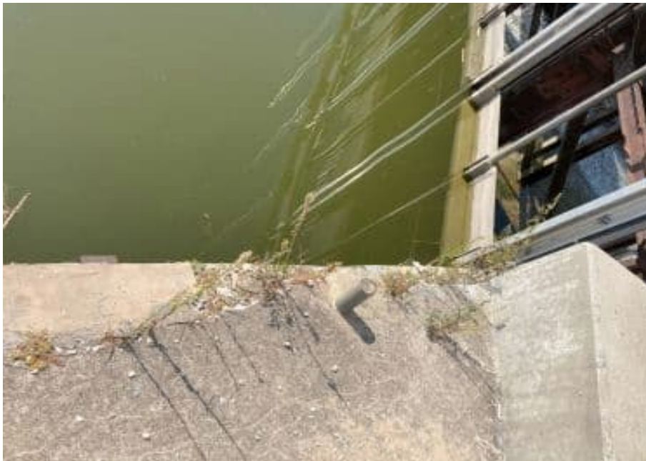
0011409092436 Chipped concrete on edge of North dam RT U/S abutment
