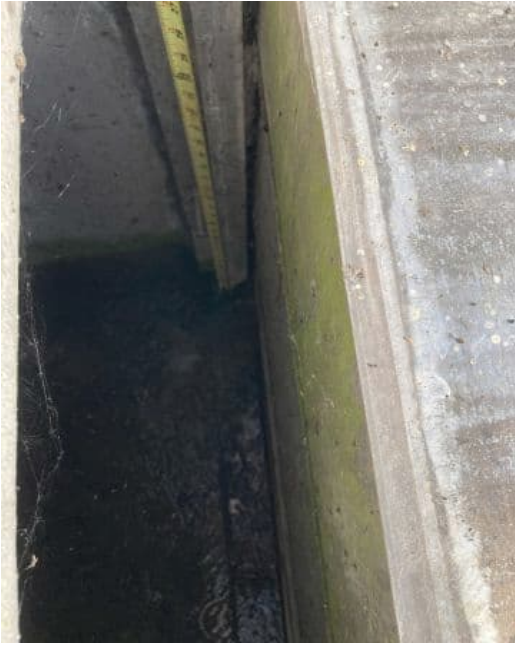
0011409092455 Slight leakage of stop logs on RT side of LT box culvert
