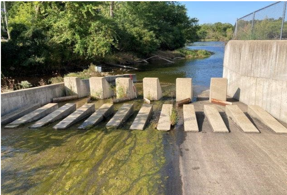
0011409092458 Looking D/S at South dam tailrace energy dissipation blocks
