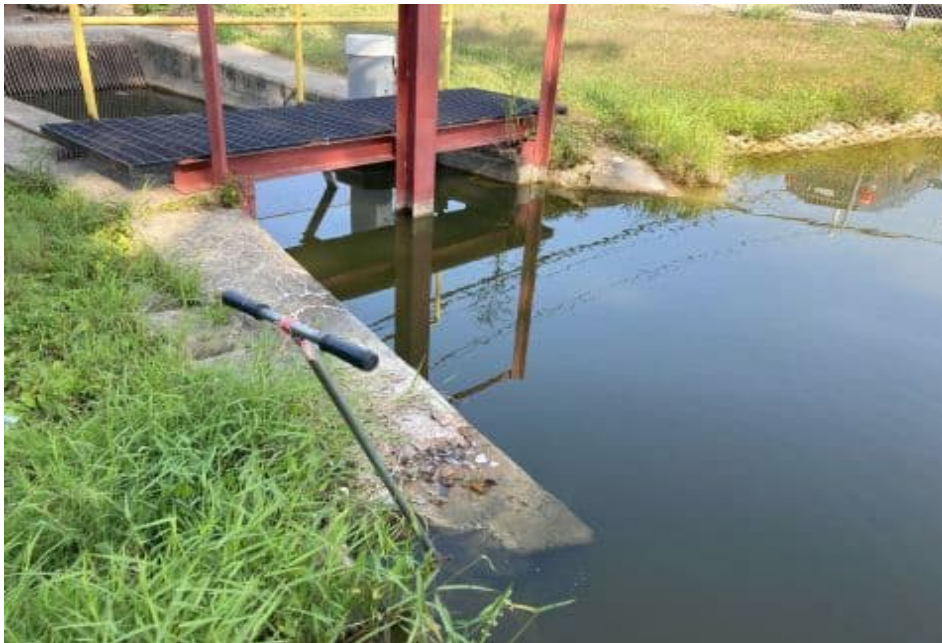
0011409092468 Concrete on South dam LT U/S powerhouse headrace abutment in disrepair
