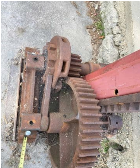
0011409092466 Replaced bolts on gate. Second bolt partially visible at opposite end of gate
