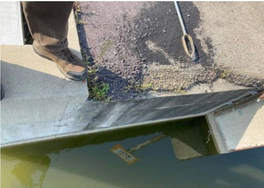
0011409092456 Asphalt patch at edge of pier at south dam inlet of box culverts
