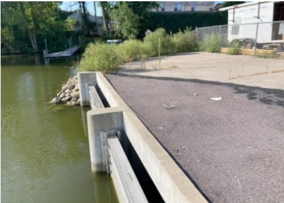
0011409092450 Stop logs at South Dam box culverts
