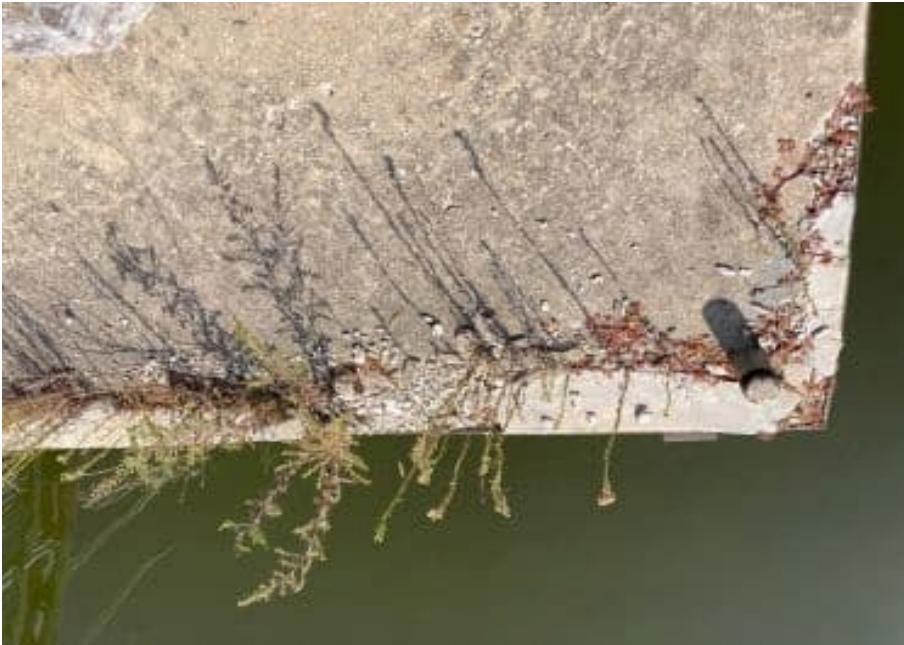
0011409092437 Chipped concrete on North dam RT U/S abutment
