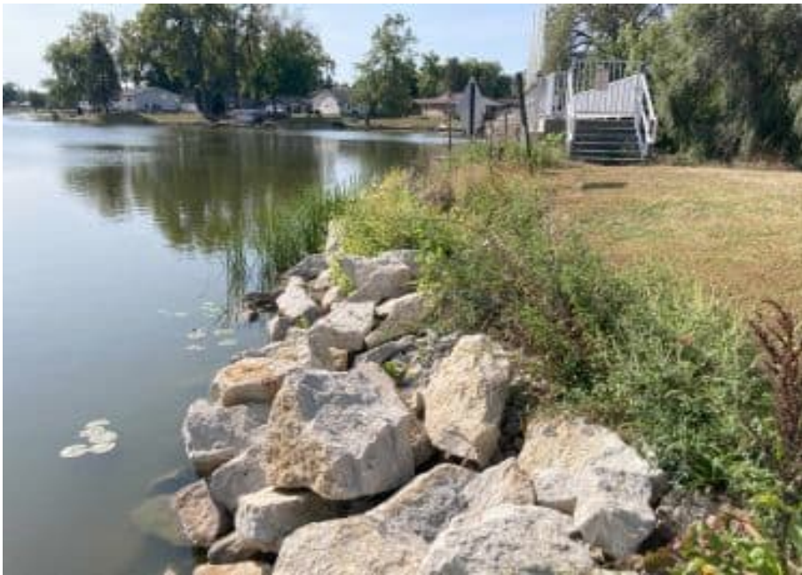
0011409092420 Looking south at riprap on North dam RT embankment U/S side
