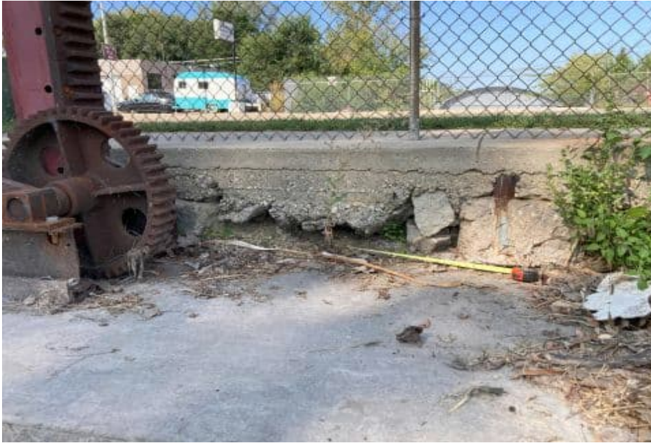
0011409092465 Retaining wall at South dam headrace in need of repair
