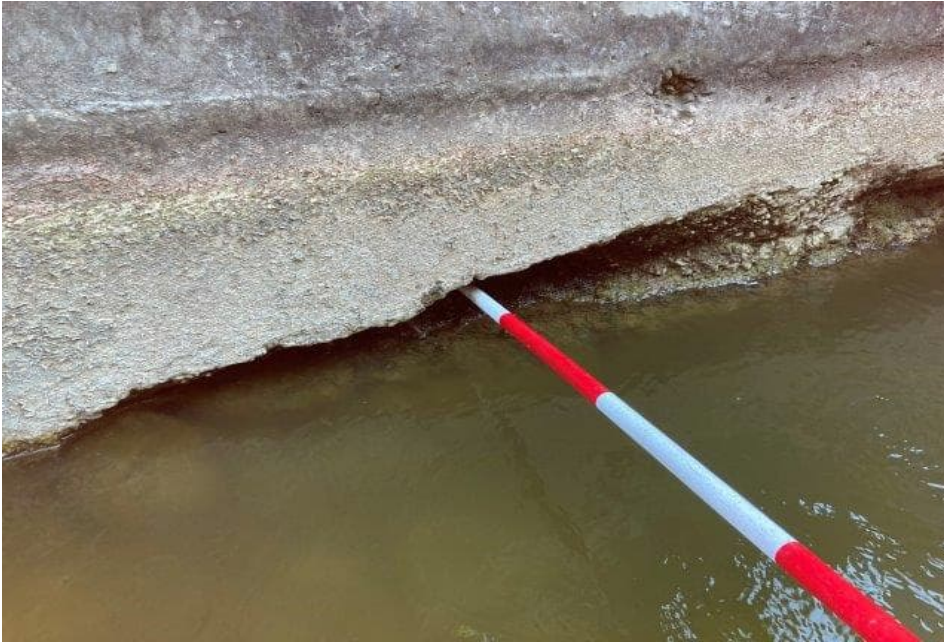
0011409092475 Missing concrete on RT wall of South dam Powerhouse tailrace
