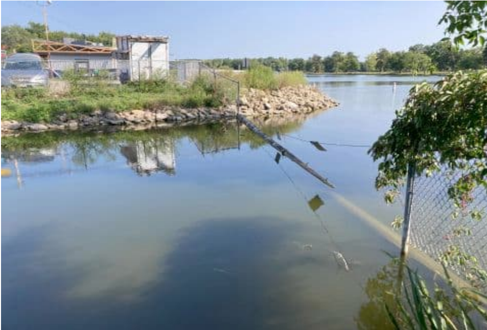
0011409092469 Debris log U/S of South dam powerhouse headrace. LT side submerged
