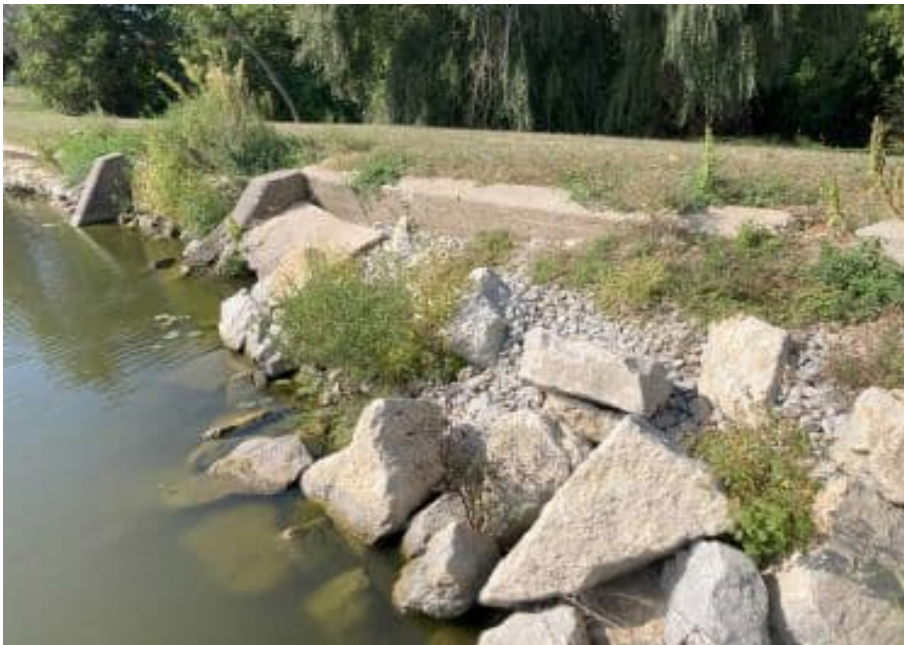
0011409092416 Looking south at North dam LT embankment failing wall on U/S side just south of LT abutment. Retaining wall in need of repairs.
