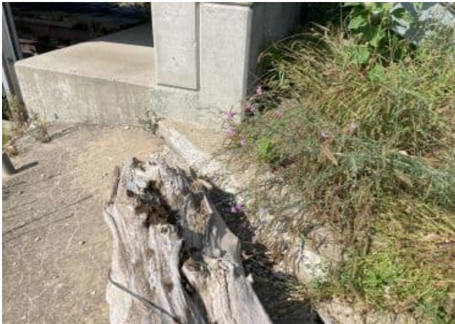
0011409092438 Chipped concrete on North dam RT U/S abutment
