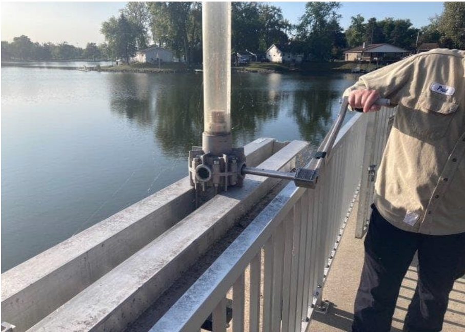
0011409092441 Hand crank gate operation for North dam
