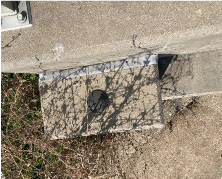
0011409092401 Benchmark on LT U/S abutment of north dam
