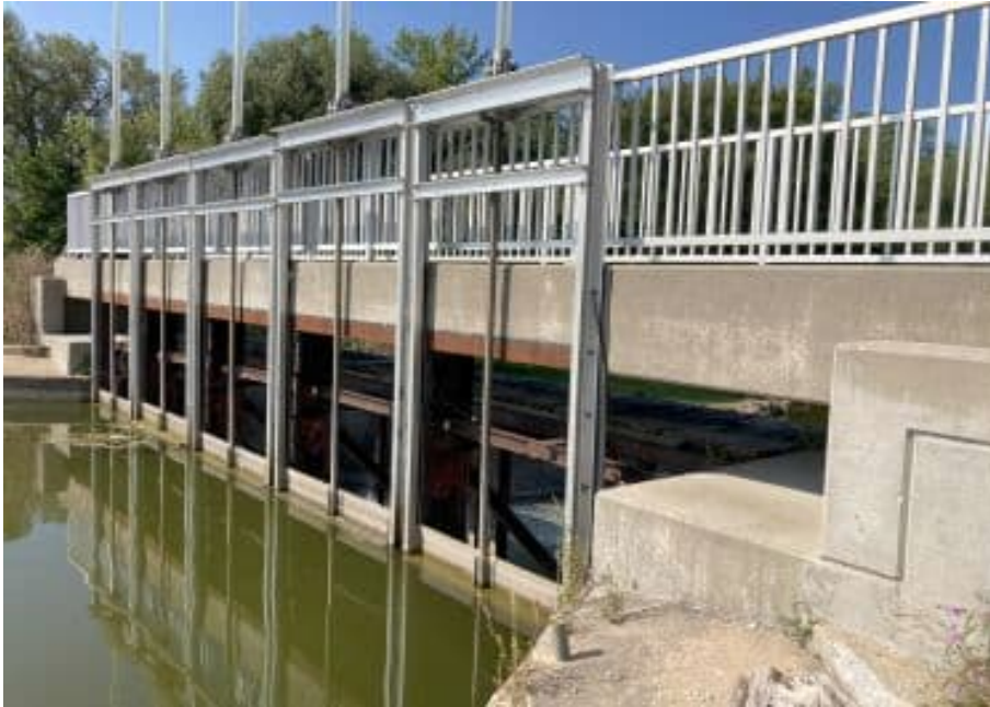
0011409092421 Standing on RT U/S abutment of north dam looking toward LT abutment. Frames and stems in good condition.
