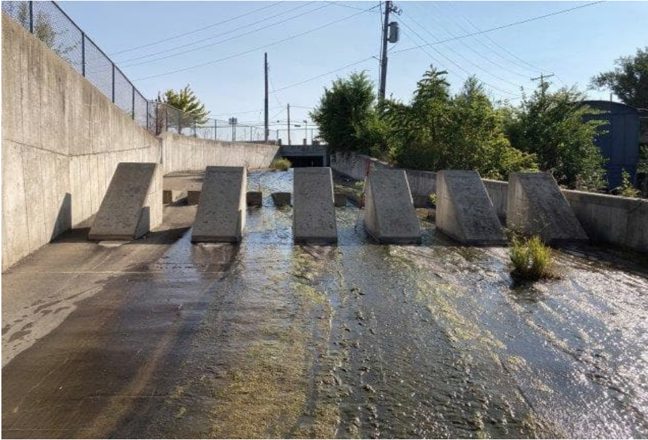
0011409092457 Looking U/S at South dam tailrace energy dissipation blocks
