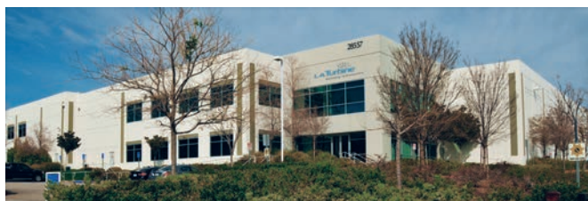
L.A. Turbine — Headquarters Valencia, CA USA
