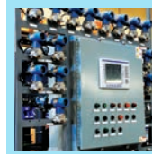
Instrumentation/Control System upgrade to integrate PLC.
