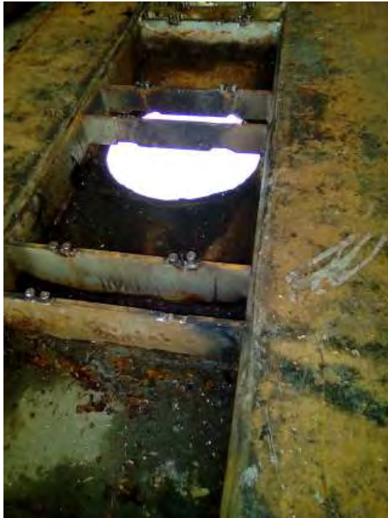
Photo 5 Skid plate structure with bridging plate removed
