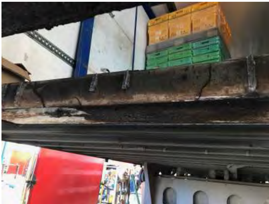
Photo 6 Crack in crossmember with skid plate removed
