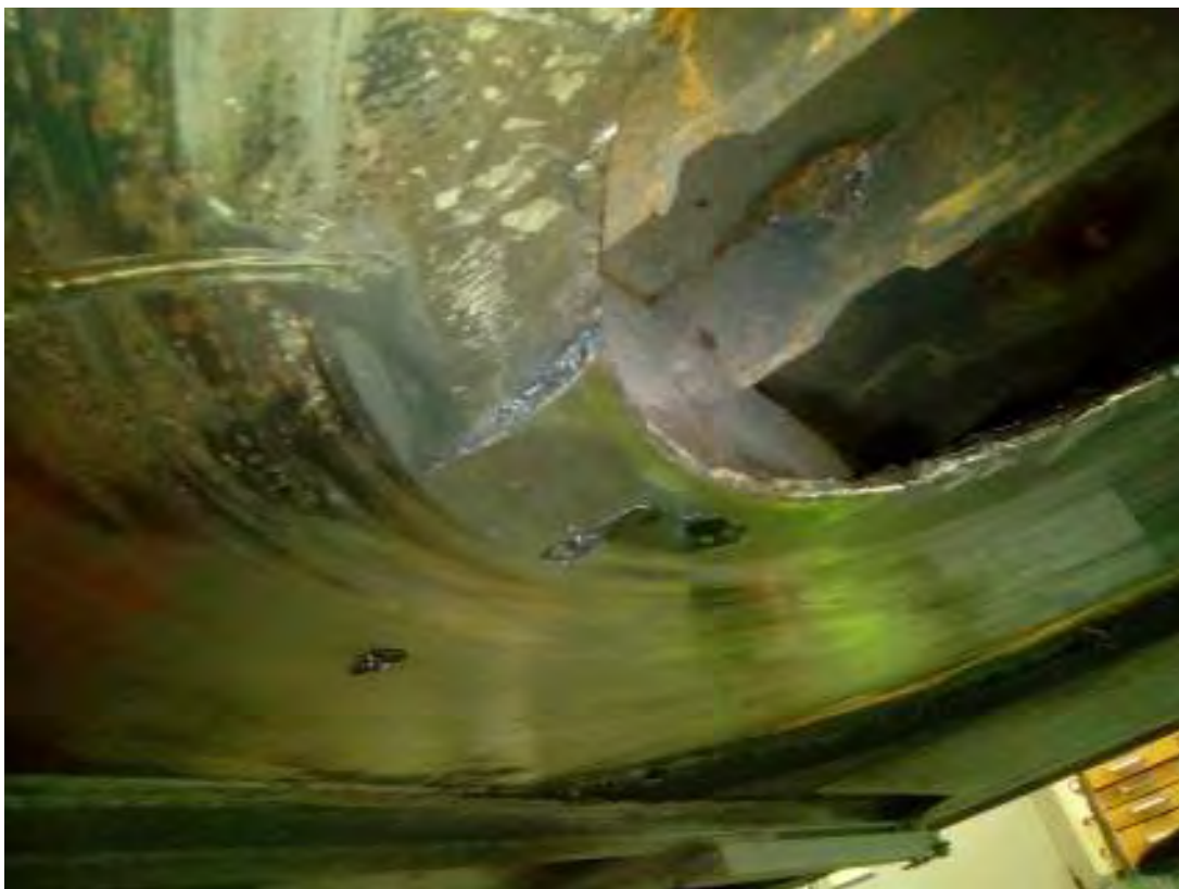
Photo1 Skidplate at initial viewing, following cleaning. View is to the rear of the trailer
