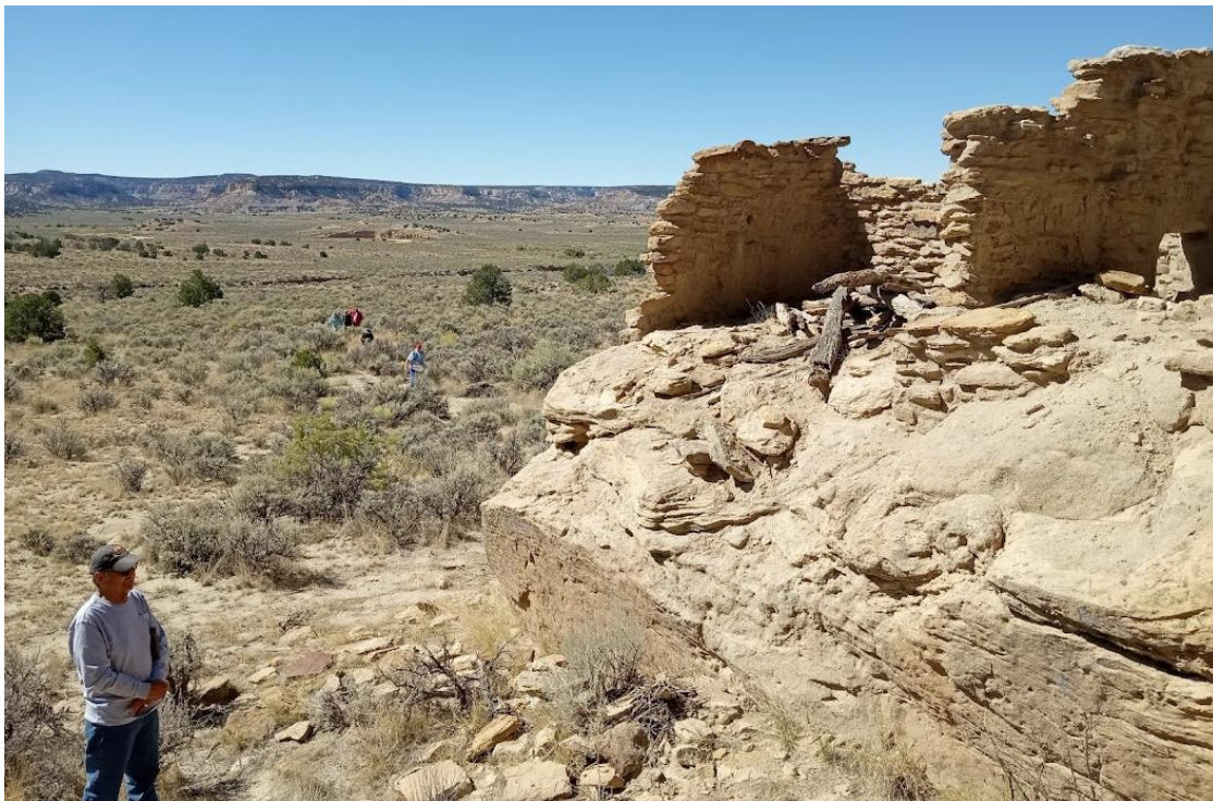
Roy Dan contemplating the completed stabilization work at Twine House.
