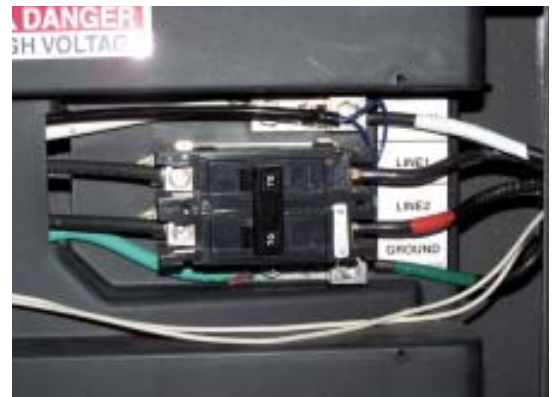
Figure 5. Since the load center in the existing panel was hard-bussed to the meter (left), the author rerouted the existing circuit wires to an electrical gutter (at bottom of photo), where he spliced them to new wires that run to a new load center on the left. A whole-house transfer switch (below left) is inside the building on the other side of the wall. The large wires on top go to the utility via the main service disconnect in the existing panel, the large pair at the bottom go to the new load center, and the wires in the conduit go to the generator, where they connect to the generator's breaker (below).
