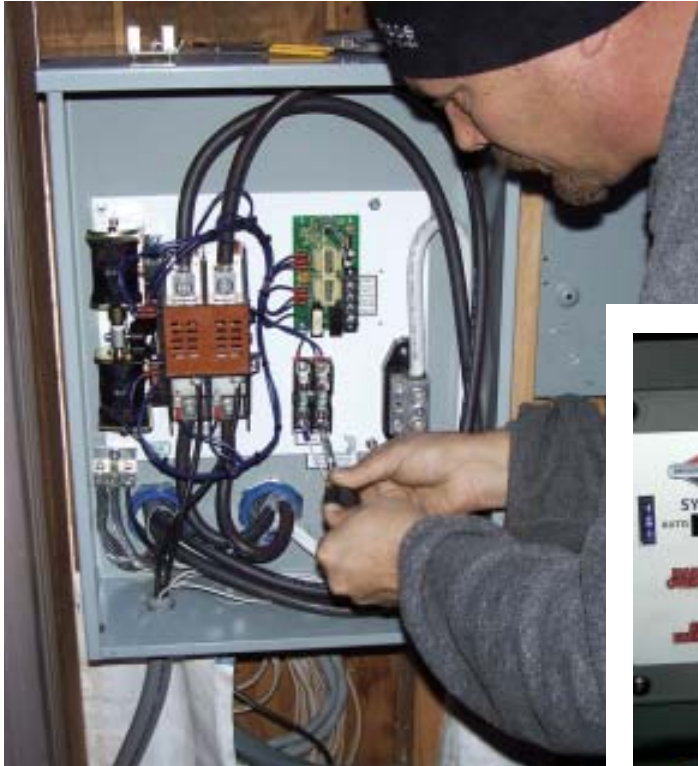
Figure 3. At left, the electrician attaches a white control wire to a fuse block connected to the electronic controller above. The controller tells the generator and the whole-house transfer switch — the device with large black wires coming out of it — when to operate. At the generator (below), the control wire is screwed to a terminal on the system control panel.
