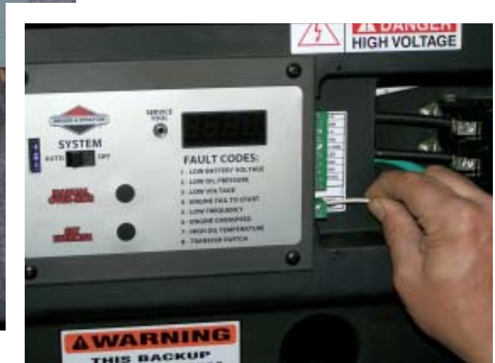
Figure 3. At left, the electrician attaches a white control wire to a fuse block connected to the electronic controller above. The controller tells the generator and the whole-house transfer switch — the device with large black wires coming out of it — when to operate. At the generator (below), the control wire is screwed to a terminal on the system control panel.
