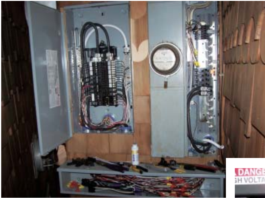
Figure 5. Since the load center in the existing panel was hard-bussed to the meter (left), the author rerouted the existing circuit wires to an electrical gutter (at bottom of photo), where he spliced them to new wires that run to a new load center on the left. A whole-house transfer switch (below left) is inside the building on the other side of the wall. The large wires on top go to the utility via the main service disconnect in the existing panel, the large pair at the bottom go to the new load center, and the wires in the conduit go to the generator, where they connect to the generator's breaker (below).
