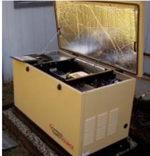
Figure 1. Most residential generators are air-cooled and burn propane or natural gas. A small standby system might have a 7-kw generator (above), while a large one might have a 13-kw unit (the minimum size for a whole-house system). This whole-house system has a 16-kw generator (right).
