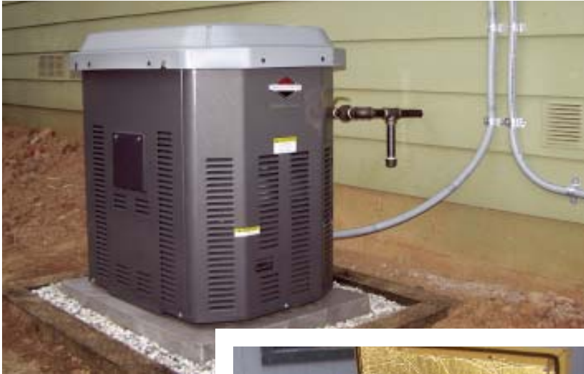
Figure 1. Most residential generators are air-cooled and burn propane or natural gas. A small standby system might have a 7-kw generator (above), while a large one might have a 13-kw unit (the minimum size for a whole-house system). This whole-house system has a 16-kw generator (right).
