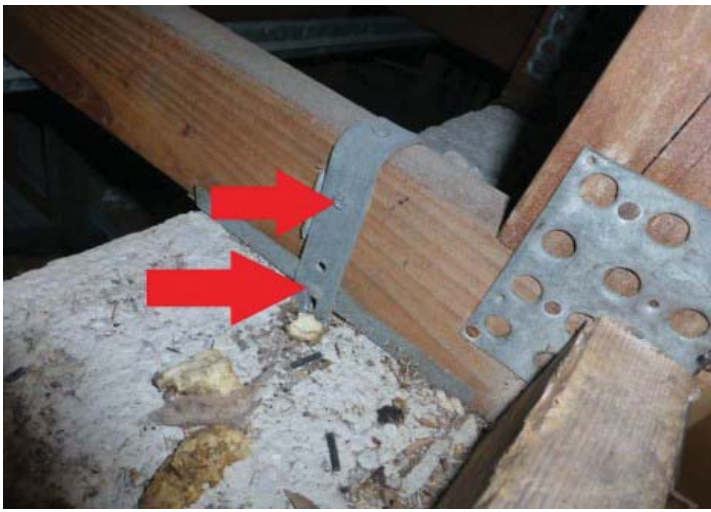
#4 ROOF TO WALL ATTACHMENT FACE SIDE
