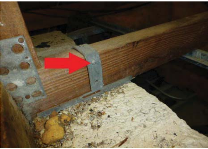
#4 ROOF TO WALL ATTACHMENT OPPOSITE SIDE
