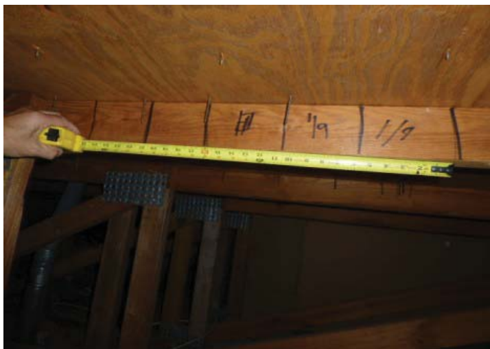
#3 ROOF DECK ATTACHMENT 6" X 6" NAIL SPACING
