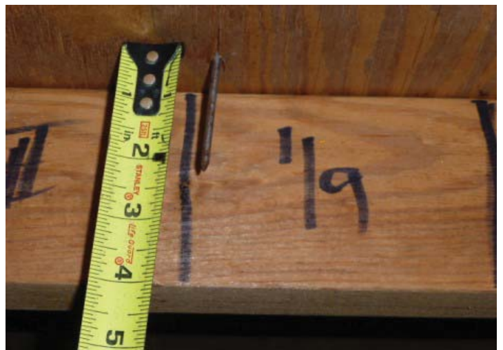
#3 ROOF DECK ATTACHMENT 8d NAILS
