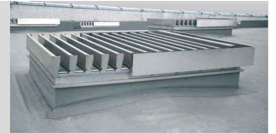
Louvre Roof Mounted Unit
