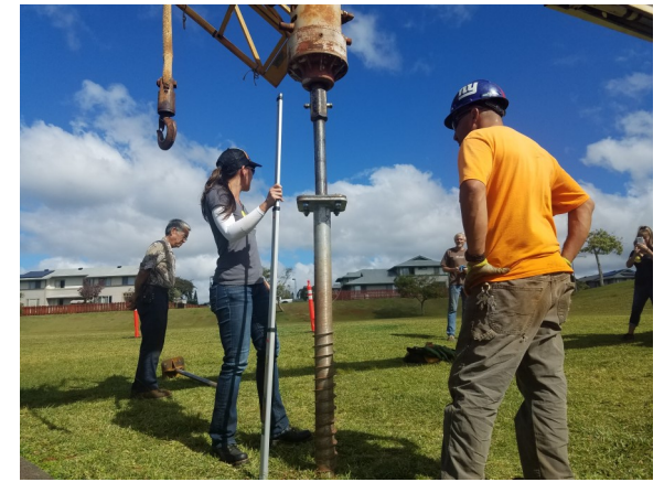
Drilling the Ground screw
