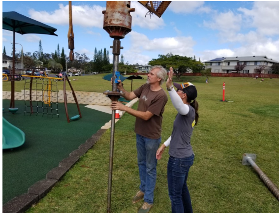
Driving a leveled drill bit to guide the ground screw.
