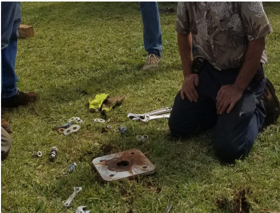
Ground screw flush with earth, ready for pole and fixture installation.
