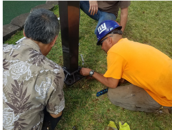
20'x5" Square Pole secured to ground screw flange.
