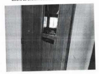
Interior Doors – The interior doors are all wooden and look aged. The picture on the left has a door that has a round door handle. This should be switched to a latch door to make steps towards ADA compliance.
