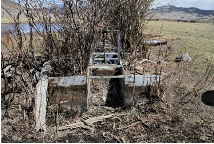
Headgate looking downstream
