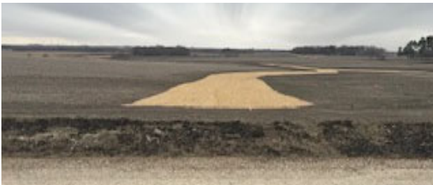
Grassed waterway with erosion blanket
