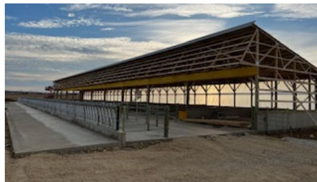
Ag Waste System
