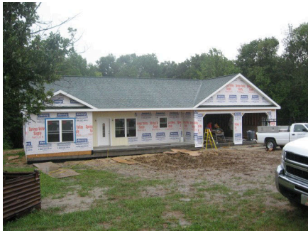
The "McIntosh Home" underway
