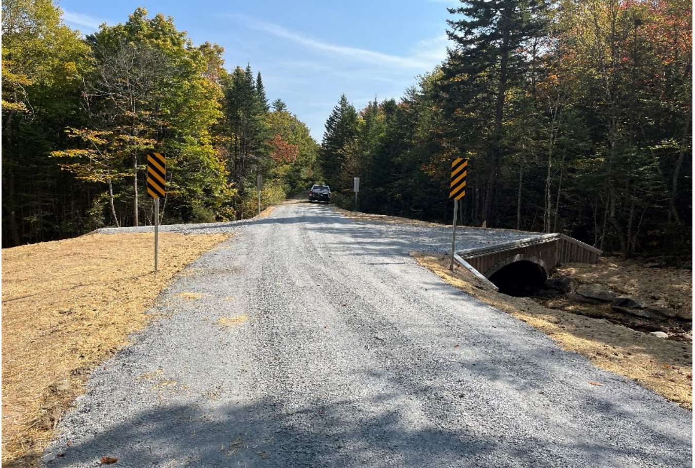
Construction of an aquatic organism passage culvert replacement on Forest Road 73 in Woodford, VT. USDA Forest Service photo.
