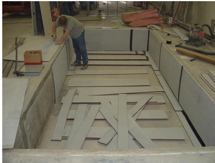
ADC Vibration Isolation Vault under Construction
