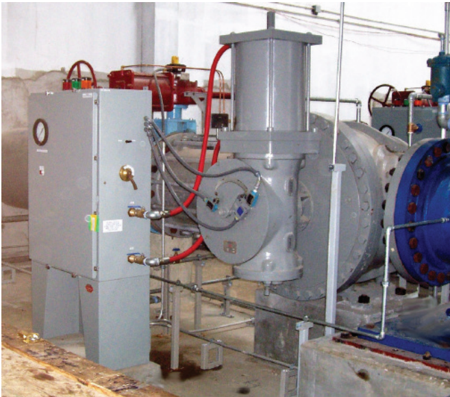
Chilibre Water Plant, Panama City, Panama — One 24" Rotovalve with hydraulic cylinder and hydraulic power unit
