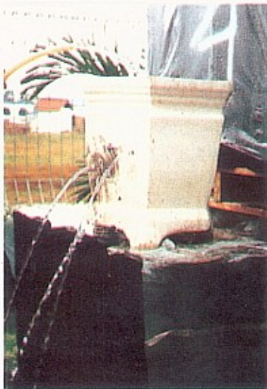
Renderoc Plug being held in place to completely stop the flow of water.
