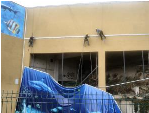
TS44 - Large non-rectangular frame. Installation of the printed graphic.
