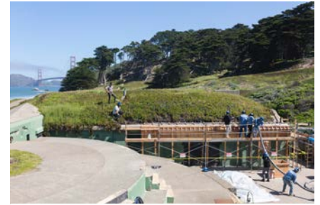
Work site; Golden Gate Bridge in background
