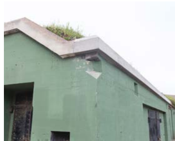
After: Repairs complete
