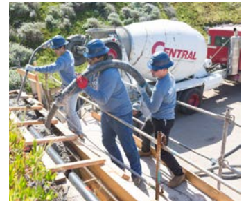
In Progress: concrete placed via pressure pumping
