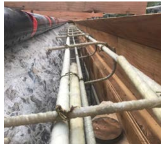
In Progress: Advanced technology glass fiber composite reinforcing for increased durability
