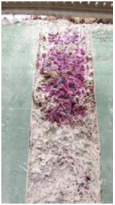
Concrete carbonation testing
