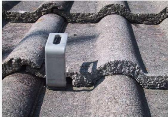
Tiles or slates removed for fixing a mounting bracket should be re-attached to include a means of mechanical fixing.
