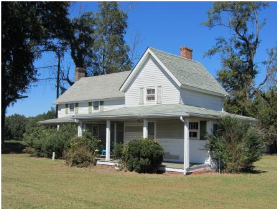
Figure 114. NCDOT Survey #49, Huffines House (GF-8207), 6021 Burlington Road, Guilford County, original core on left with addition on right with wraparound porch, looking northwest.
