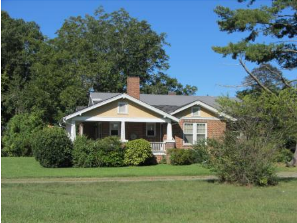
Figure 108. NCDOT Survey #26, Hoffman House (GF-8187), 6805 Burlington Road, Guilford County, east gable end, looking west from Woodard Road.
