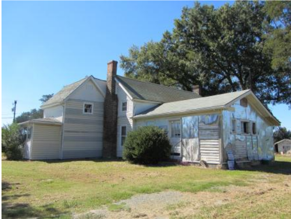
Figure 113. NCDOT Survey #49, Huffines House (GF-8207), 6021 Burlington Road, Guilford County, main core with east addition and north wing, looking southwest.
