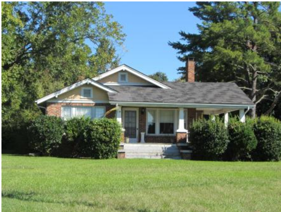
Figure 107. NCDOT Survey #26, Hoffman House (GF-8187), 6805 Burlington Road, Guilford County, south façade, looking north from US 70.
