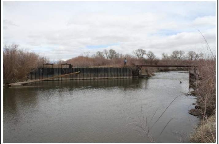
Headgate and diversion dam
