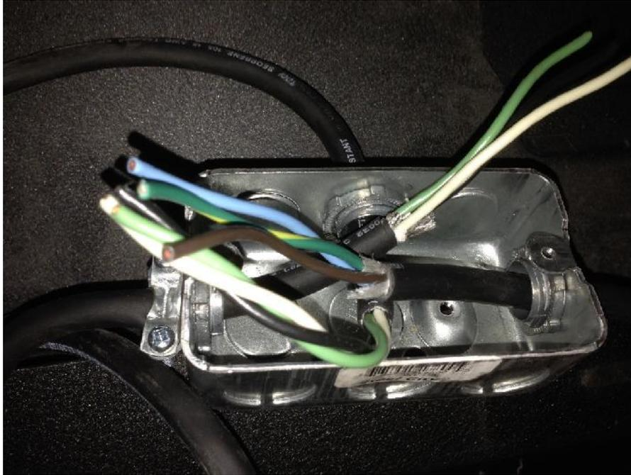
We made the connections with wire nuts and put the box cover on. The box fits in the monitor support wireway nicely and is out of view. Daily hours:  $9 + 16 = 25$ . Job hours:  $49 + 82 = 131$ .
