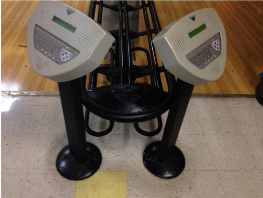
The settee area is concrete with a 16" drop at the start of the approach for the lanes footprint. Here (below) is a picture taken from under the ball storage rack toward the settee area showing the solid concrete settee area which has two conduits for running the bowler's terminal cables to each of the bowler's terminal pedestals:
