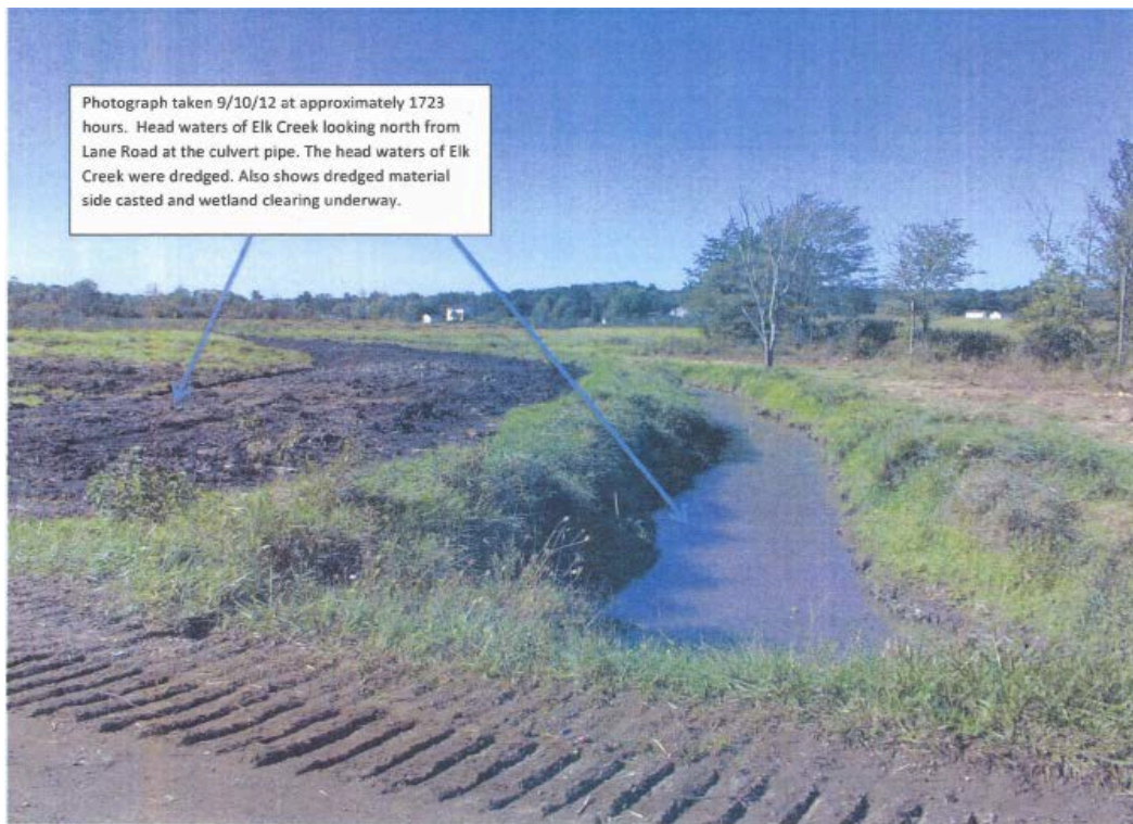
Figure 14. September 2012 photograph from Marsh Site inspection by Smolko; Elk Creek from Lane Road looking downstream (north) showing disturbed soils and side-casting from dredging Elk Creek.
