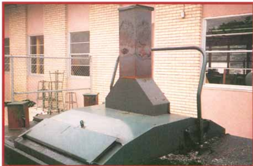
The Afterburner burns off 81 percent of the particulate matter and 77 percent of the hydrocarbons from the fumes.
