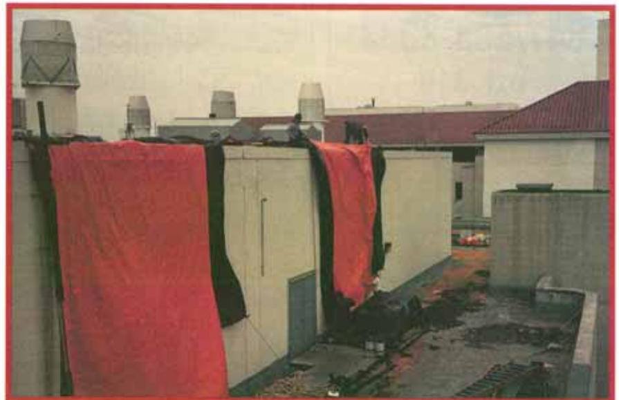
Louvers on building walls or intakes on rooftop mechanical equipment can be temporarily concealed with polyethylene (plastic) sheeting to avoid odor infiltration into the building.
