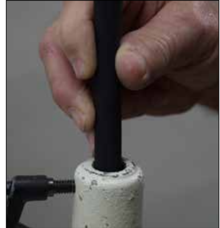
Post hole 1413. Clean inside the post hole with rolled up non-woven abrasive.
