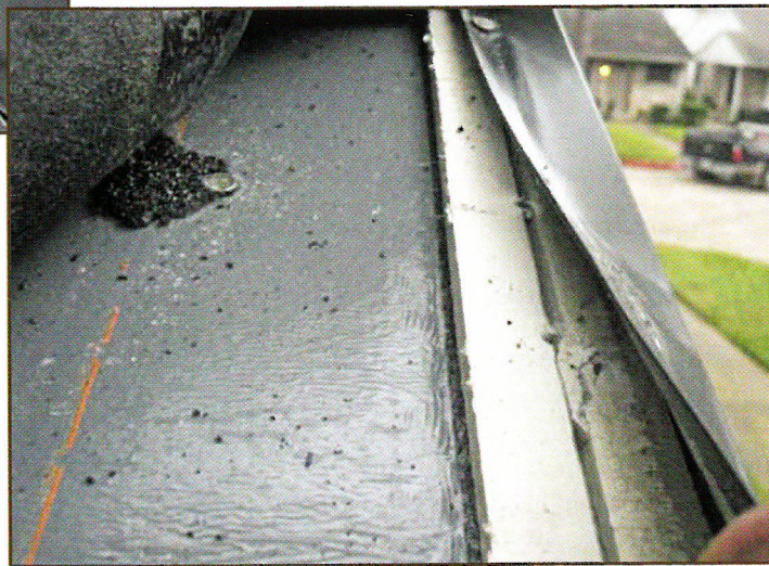
Figure 19 – Fasteners for rake flashing installed in joint between fascia cement boards.
