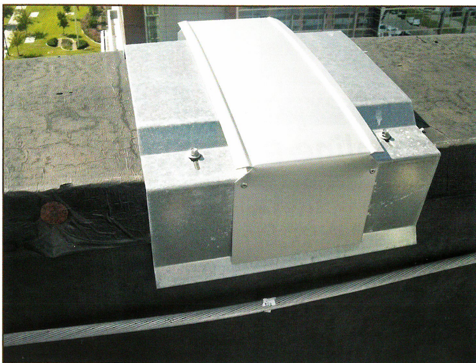
Figure 17 – Typical cleat/chair for coping.
