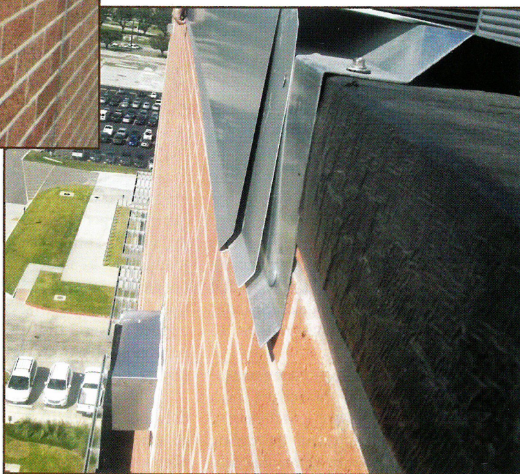
Figure 16 – Drive pin installed in face of cleat.
