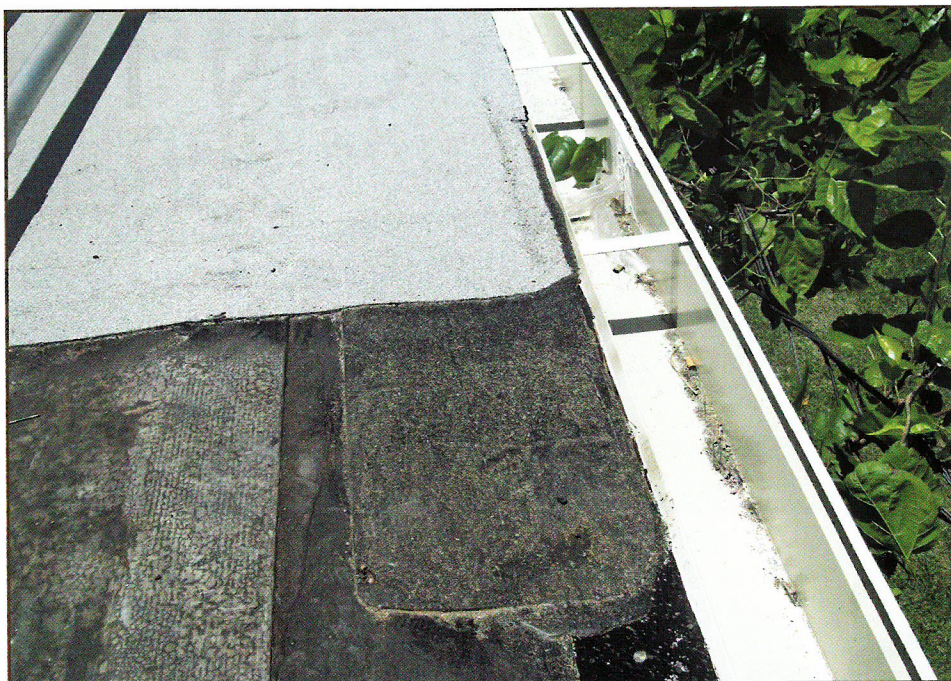
Figure 4 – Metal edge, strip-in, and cap sheet.
