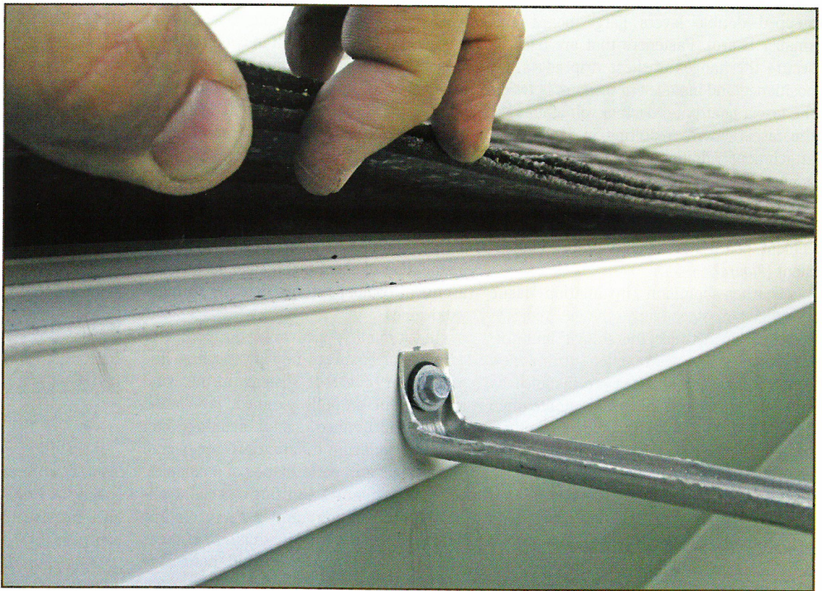
Figure 20 – Gutter spacer fastened into face of drip edge; also note no visible fasteners in flange of drip edge.
