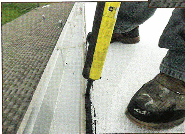
Figure 5 – Applying edge sealant.
