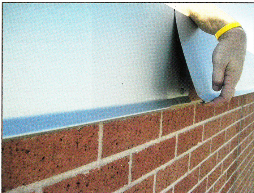
Figure 15 – Fascia of coping not engaged to cleat.
