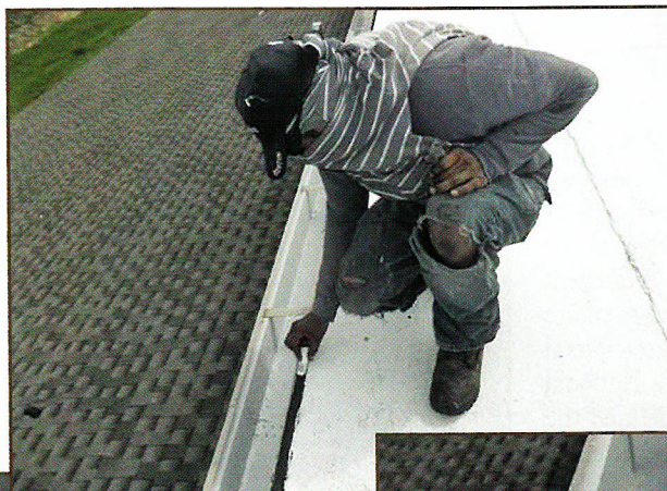
Figure 5 – Applying edge sealant.
