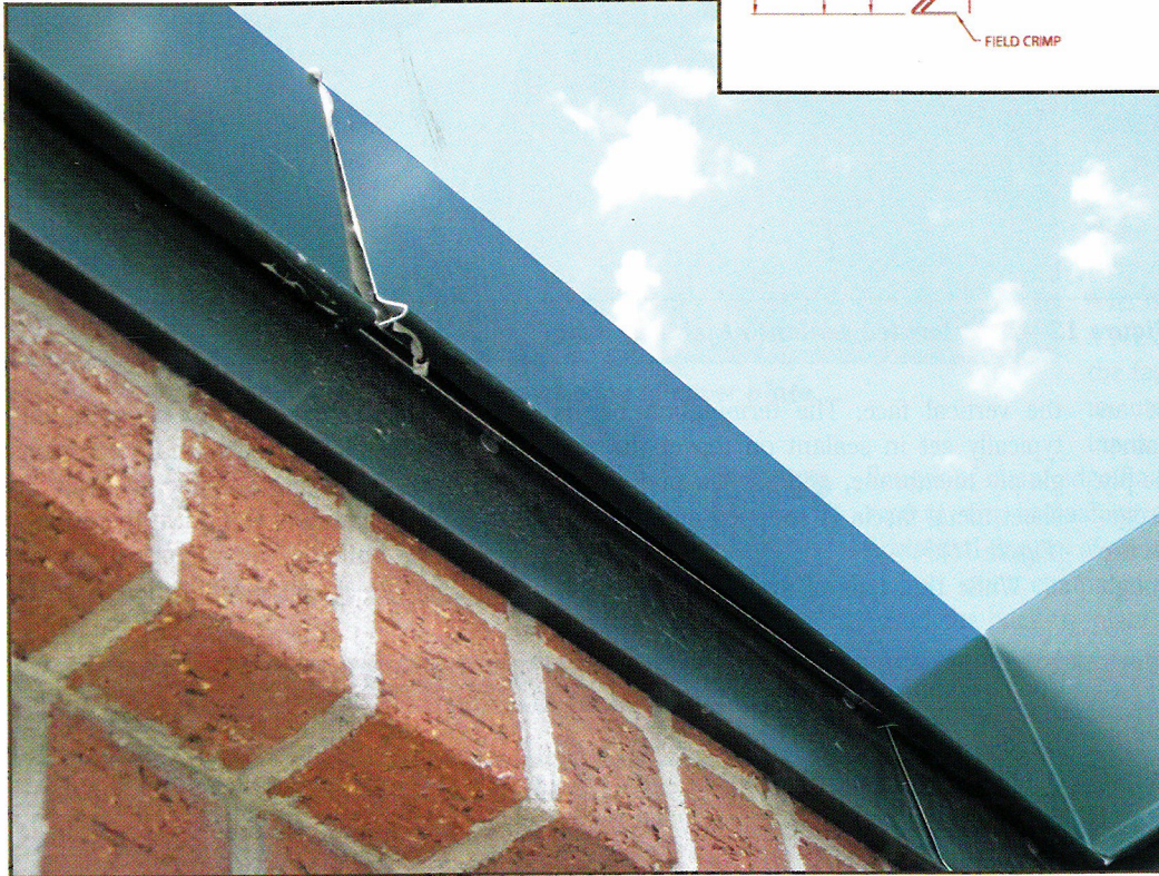
Figure 14 – Metal snap-on fascia not engaged to cleat.
