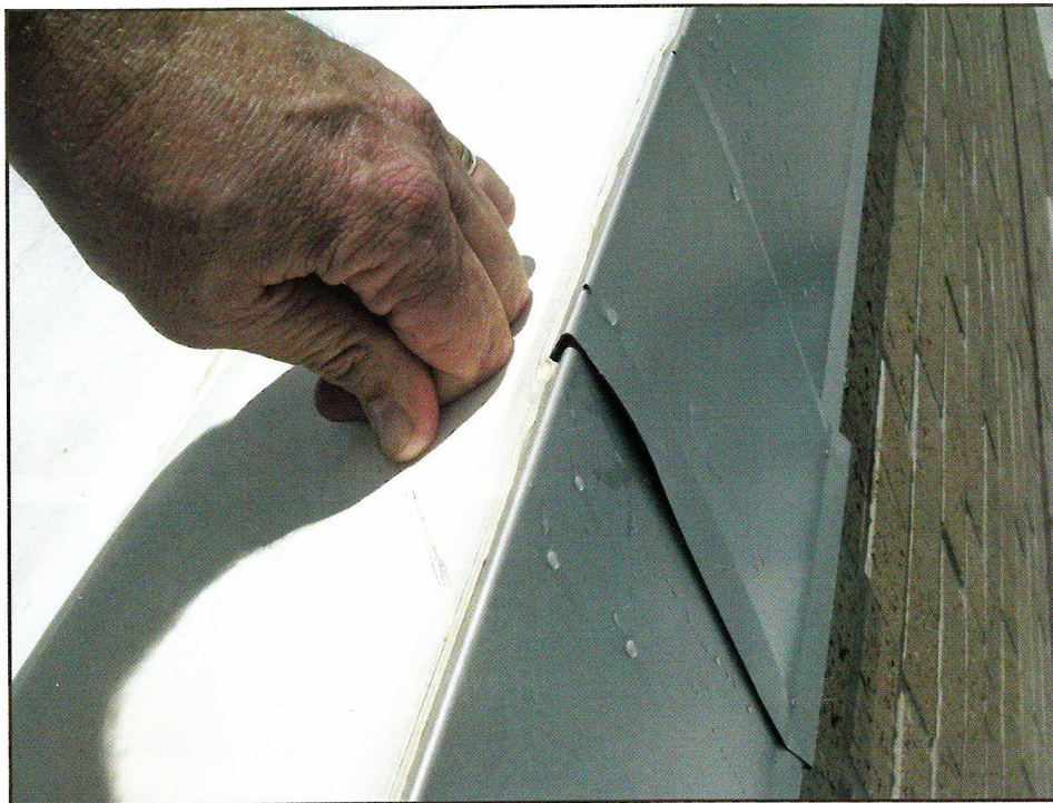
Figure 9 – Water under single-ply strip-in at edge of cover plate.
