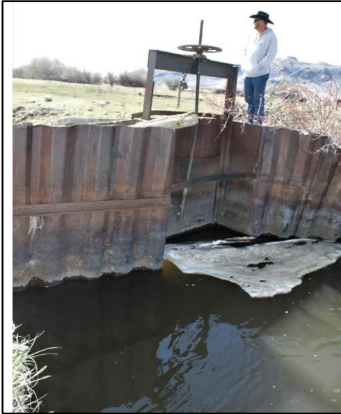
Headgate looking downstream
