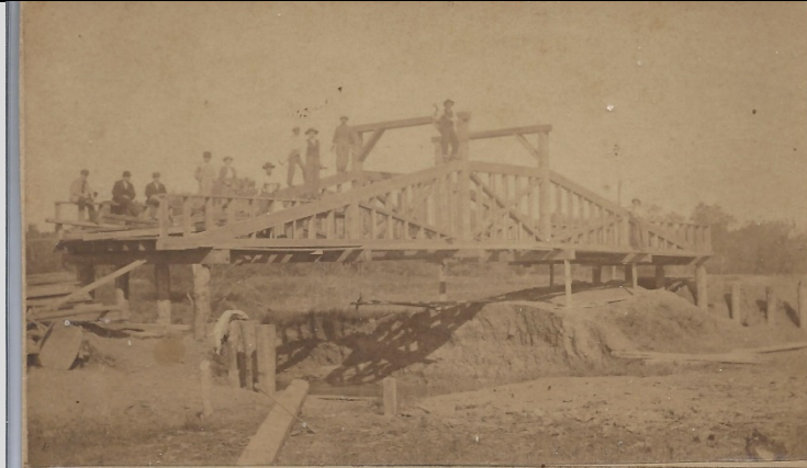
A Bridge Under Construction
