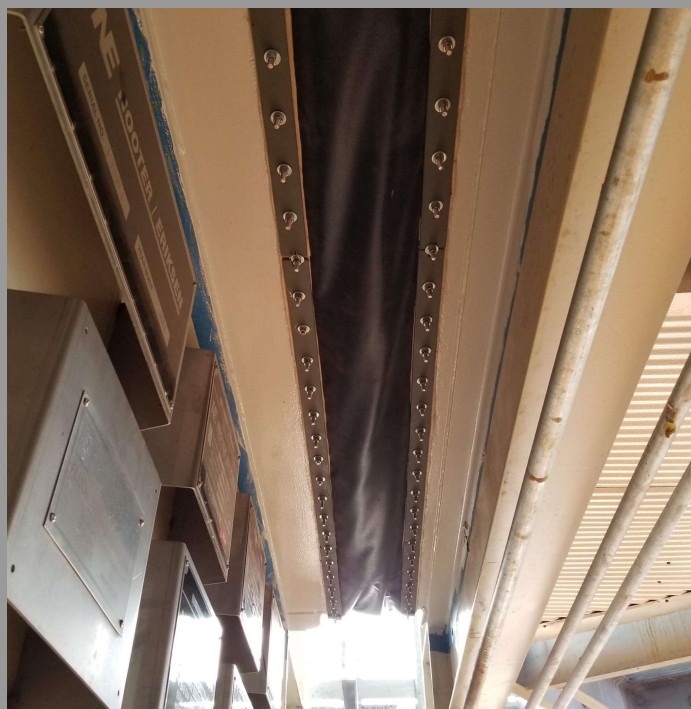
Complete Stack Seal Refurbishment
