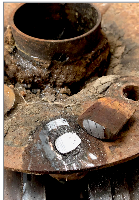
Old brake camshaft shaft sawed away
