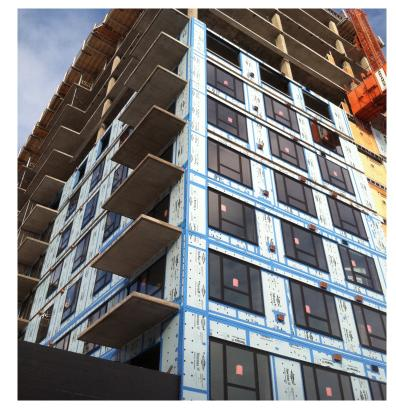
In short, the three-in-one THERMAX Wall System delivers continuous insulation, which eliminates the need for two separate production installations – an exterior sheathing and an air barrier in commercial construction. Such insulation is continuous across all structural members without thermal bridges other than fasteners and service openings.
