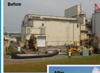
Vitrification Facility Demolition
