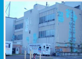
Main Plant Office Building
