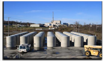
HLW Canister stored on site in Dry Cask Storage (5 canisters/cask)
