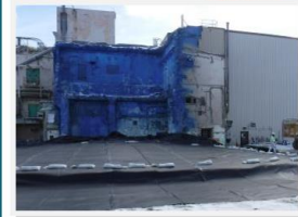
Weather protective cover installed
