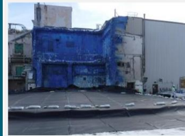
Weather protective cover installed
