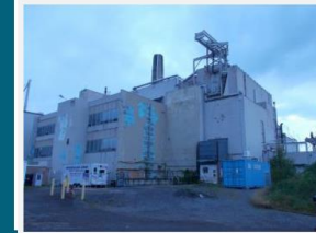
Main Plant Process Building
